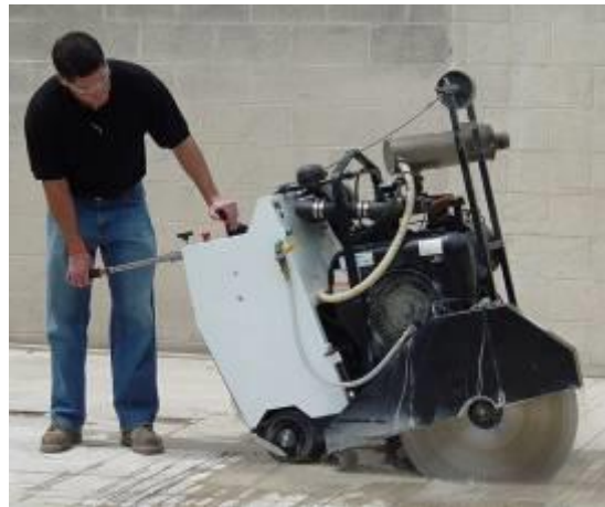
Flat saw making a cut.
