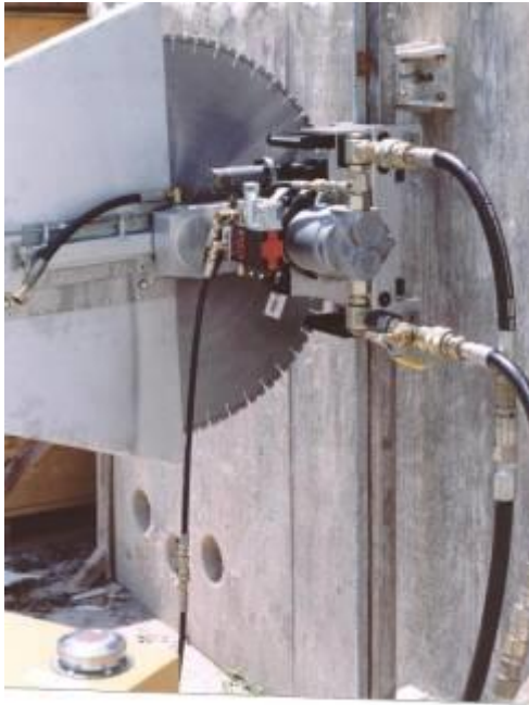
Wall saw preparing to make a cut
