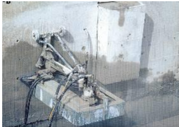
A wire saw could be used to create an opening in concrete instead of a wall saw.
