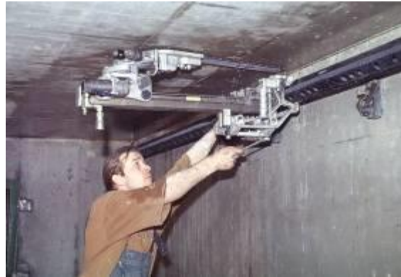
Corner cut chain saw preparing to finish the cut
