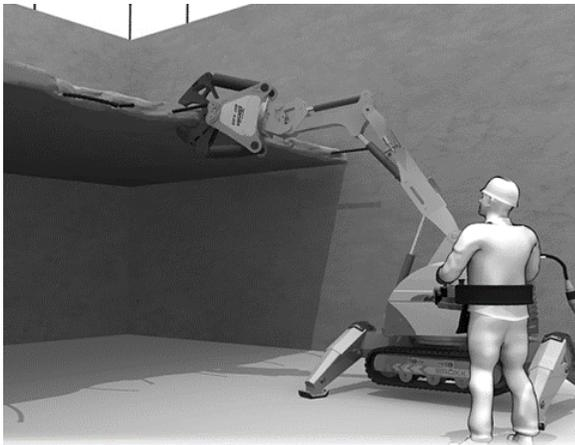
4.8 Demolishing with a crusher:
